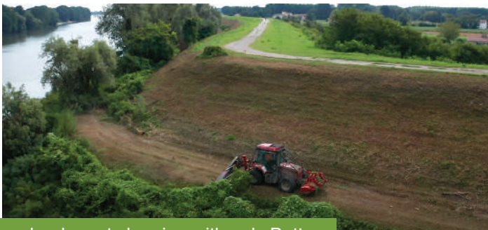
embankment cleaning with only Better
