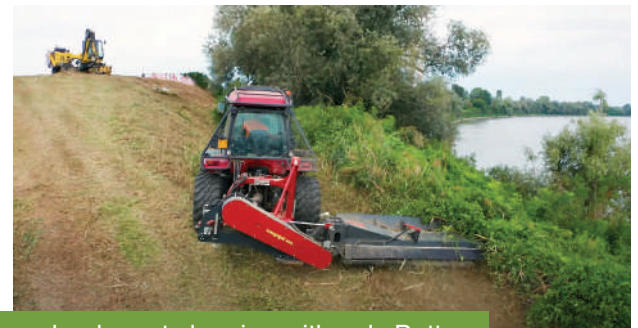
embankment cleaning with only Better
